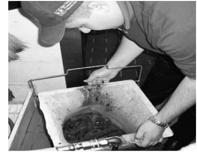
9. Raise the strainer and rest it on the center handle bar.
