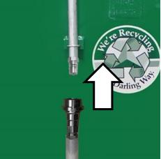
Connect the White Hose to the Grease Tank Inlet.
